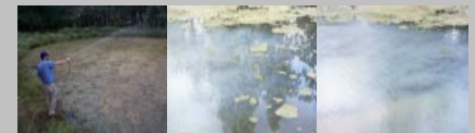
Surface application of alum solution and initial reaction of alum with water
